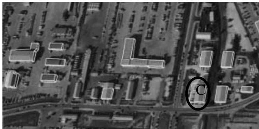
Figure 7 Section of the Motor Pool Area of Fort Hood, TX
