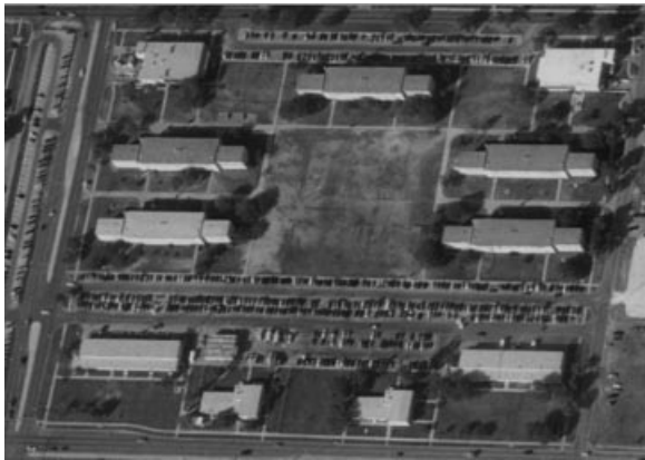
Figure 4. Barrack buildings at Fort Hood
